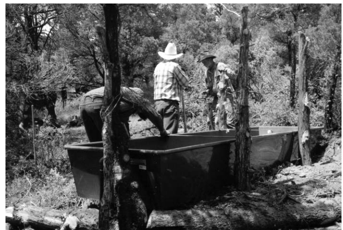
Volunteers installing watering trough in a remote area. Trough was helicoptered to site. Photo by Frank Jones.
