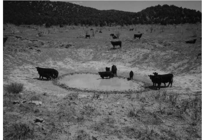
Water catchment area created with help of volunteers in Dedicated Hunter program on Pine Valley District of Dixie National Forest. To seal bottom, district employees lined pond with blue clay to retain water (lighter color). Photo by Frank Jones.
